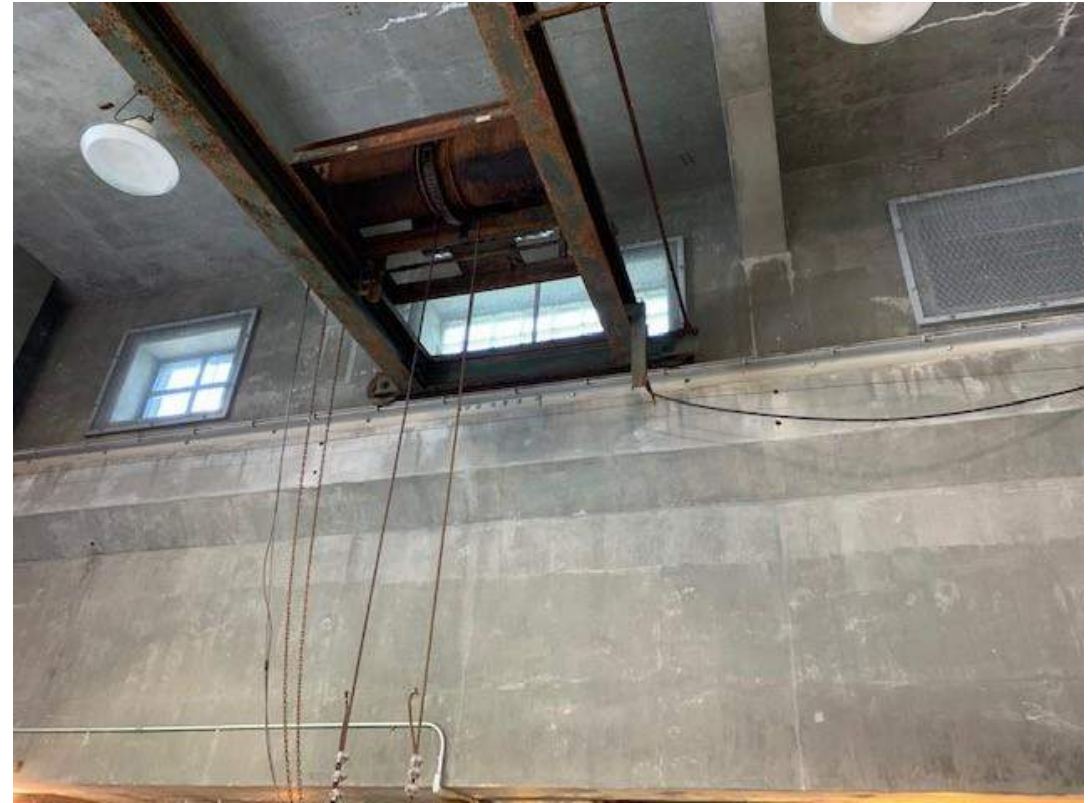
Existing Overhead Crane
