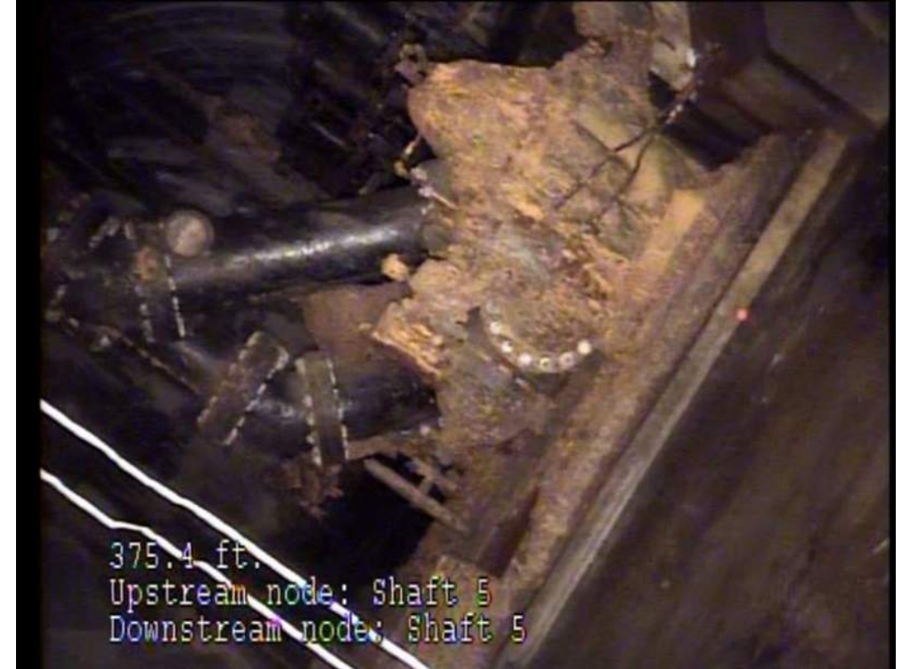
Underground pump room (abandoned with fill)
