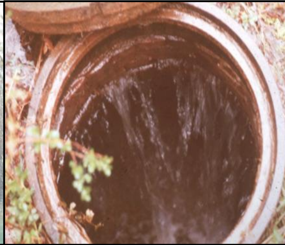
Inflow (Stormwater via direct connections)
